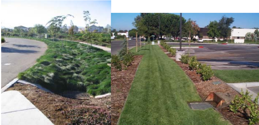
Fig. 3: A vegetated swale.
