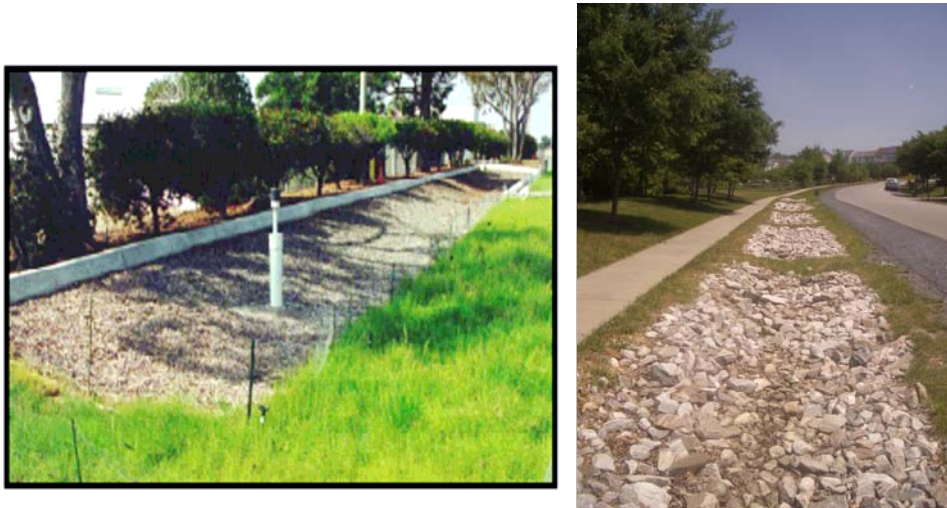
Fig. 2: An infiltration trench.
