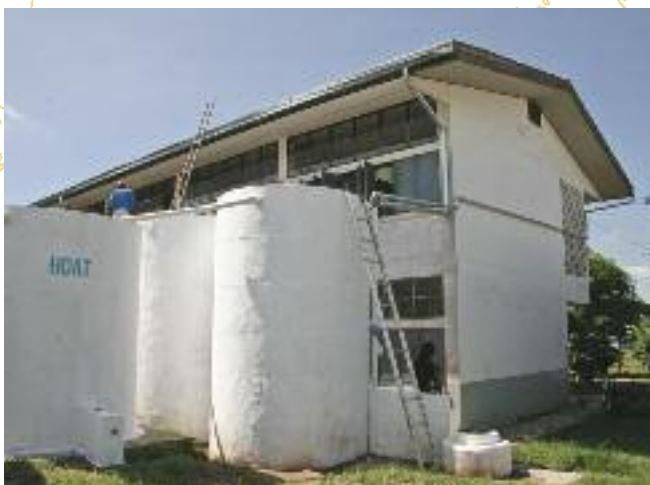
Water tanks for rainwater
